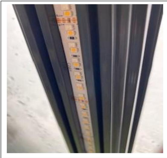
4. Feed the coloured cables under the glazing bars and along the wall plate to the required location where your connection box will be fitted. These should not be seen.
